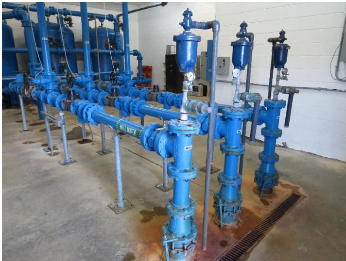
*Figure 1. Well Intakes at the Hopyard Farm Water Treatment Plant*
